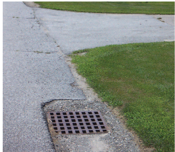
Wallingford, VT. The relative presence or absence of storm drains is one indication of how well green space is being used to manage stormwater.
