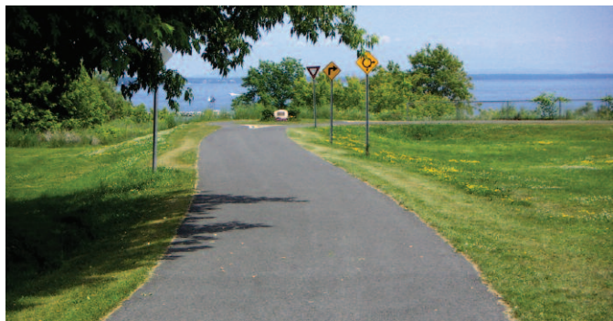
Plattsburgh, NY. Stormwater from walkways and bicycle paths often can be managed simply with a well-designed buffer.
