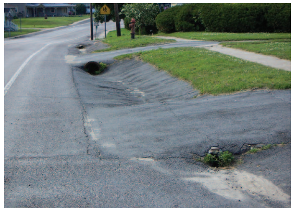
Keeseville, NY. Fast, paved ditches can be replaced with slow, vegetated swales, using drainage easements on private land if necessary.
