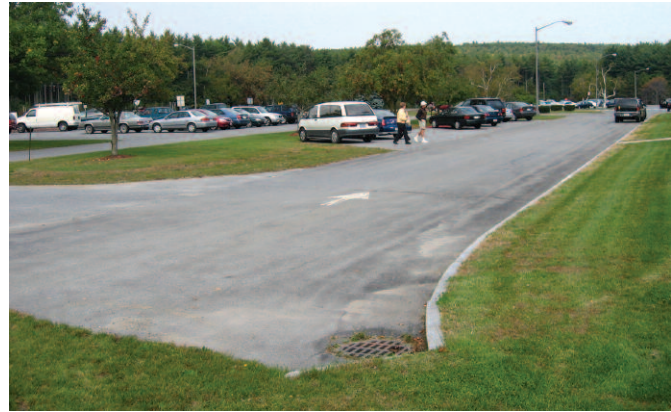
Lake George, NY. The design of this parking lot ignored the opportunity to drain stormwater to adjacent green space.
