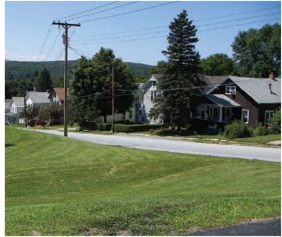
Rutland, VT. Grassed swales and other vegetated drainage channels help slow and infiltrate stormwater as it travels downhill.
