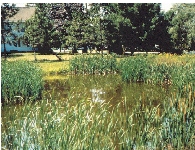
Williston, VT. Large stormwater management facilities, such as this artificial wetland, can also blend into neighborhood design.
