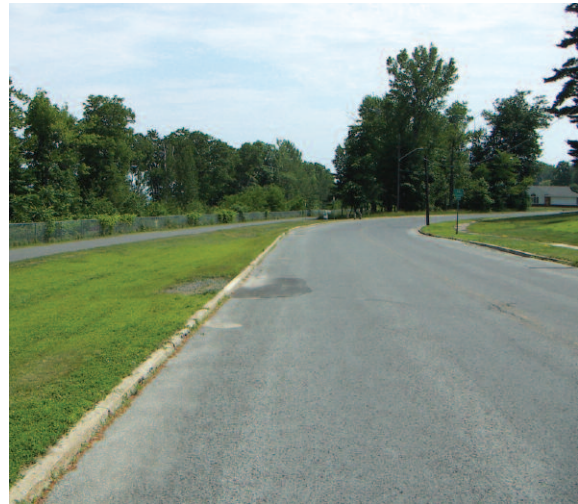
Plattsburgh, VT. Stormwater is often prevented from draining to green space by curbing or other site grading features.
