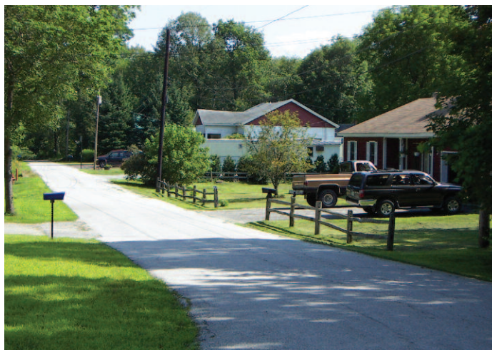
Castleton, VT. Road specifications should promote narrow roads in low-traffic neighborhoods.
